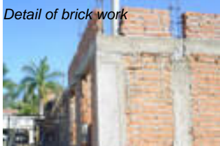
Detail of brick work
